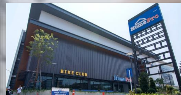
Home Pro Warehouse 3
